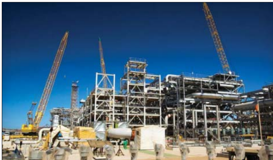
Higher labor costs forced Woodside in September 2006 to raise its project budget for Phase V expansion at the onshore gas plant near Karratha, WA, to $2.425 billion (Aus.) from $2 billion. Included is construction of a 4.2-million-tpy LNG processing train and a second loading berth. The expansion targets mid-2008 for completion. Photograph from Woodside.
