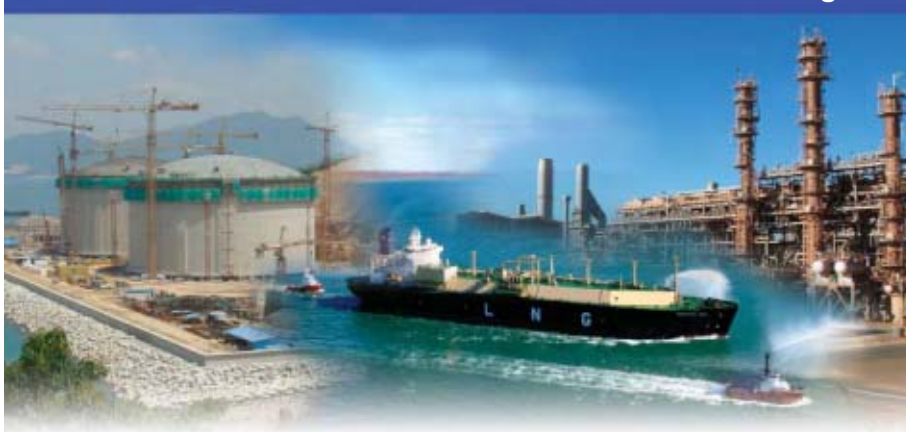
Left to right: Guangdong LNG terminal, China (photo from Guangdong Dapeng LNG Co. Ltd.); North-west Swan (photo from Woodside); Karratha gas plant, Western Australia (photo from Woodside)
